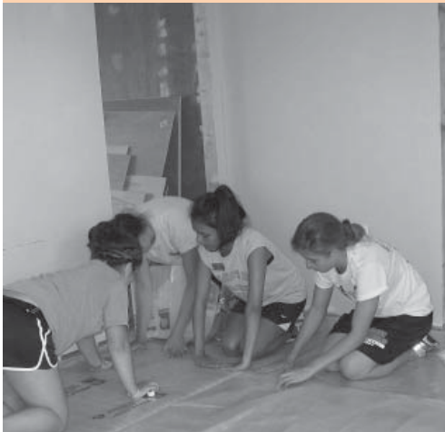
Volunteers from CND and Holy Angels install flooring
